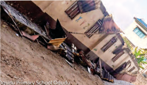
Ogudu Primary School Ogudu
